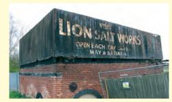
Brine was pumped to a brine tank ready to be gravity fed to the salt pans.
