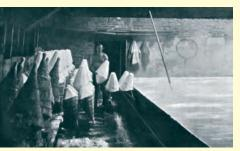
Salt was skimmed into salt moulds - originally baskets, later cooper made cones, then wooden boxes.
